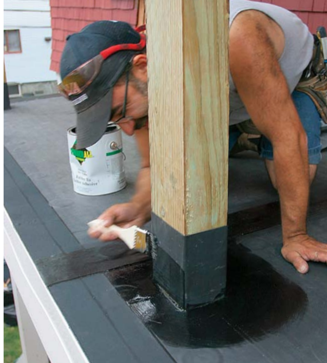
Paint on the glue. Spread splice adhesive on the roof and on the post wrap.
