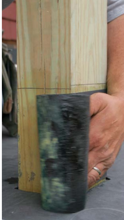
Wrap the post first. Wrapping the post with membrane provides a reliable base for gluing additional rubber for flashing.
