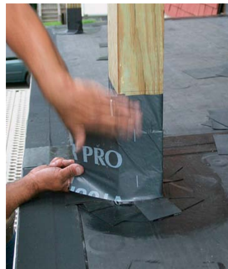
Counterflash. Once the post is fully flashed to the roof, counterflash with layers of bituminous membrane going up the post about 3 ft.
