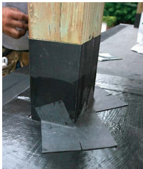
Start at the bottom. Split a scrap of rubber so it can go around the corner while lying flat on the roof. Stretch the rubber a little so the apex of the split is placed above the roof plane.
