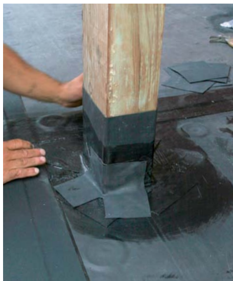
Overlap the first layer. Split a second scrap of rubber like the first. Install it to wrap the corner and splay onto the roof. The apex of its split must be on the roof so that the two apexes don't align and create a potential leak.
