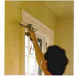
**Caulk before you paint.** Before the walls or trim is painted, a bead of paintable caulk is applied to fill the gap between the trim and the walls.
