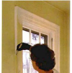
**Overlap each layer of paint.** Beginning with the primer on the trim, each coat of paint should extend slightly onto the adjacent surface, producing a cleaner line.
