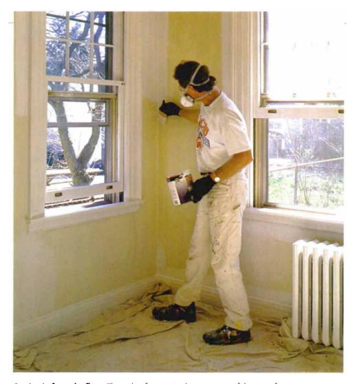
**Cutting in from the floor.** The author first cuts in the upper part of the room from a ladder, then works his way around the room, standing on the floor and cutting in.
