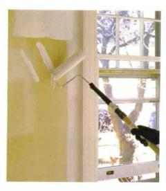
**The end of the ropes.** Ropes, or heavy lines of paint, show up when there is too much paint on the outer edges of the pad. Running the edge of the roller on the wall squeezes out the excess paint.
