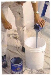
Blend all the finish paint together. Custom-mixed paint can vary in color from can to can, so all the paint is mixed together in a 5-gal. pail before it goes on the walls.
