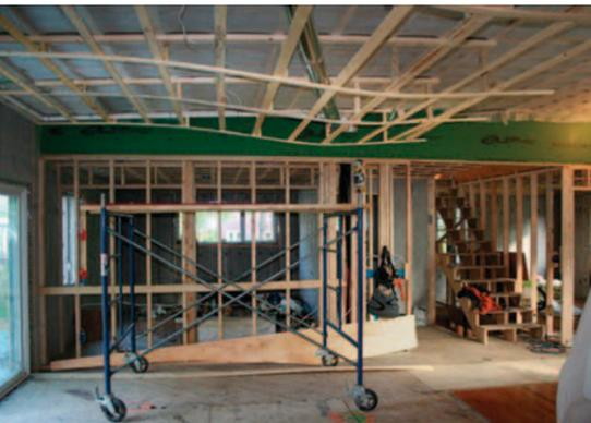
Bones of the wave. The framers used a plywood template to position strapping on the ceiling to support 16-ft. lengths of drywall. The result was an undulating ceiling that flows over the bright, airy kitchen. All appliances were salvage finds and kept costs low.
